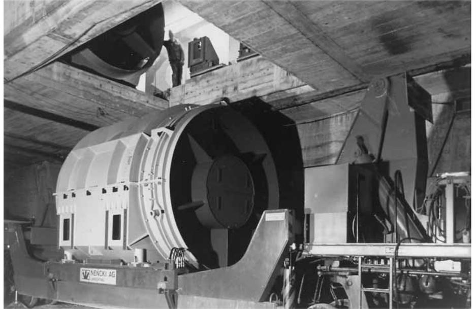
Fig. 6: Axial-flow fan during installation in the fan house
