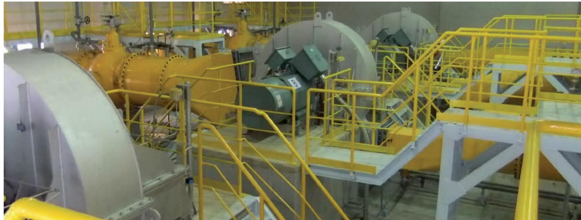
LD booster fans downstream of a gasometer in a steel mill. The housings are made gas-tight because of the high proportion of CO gas in the extracted gas.
